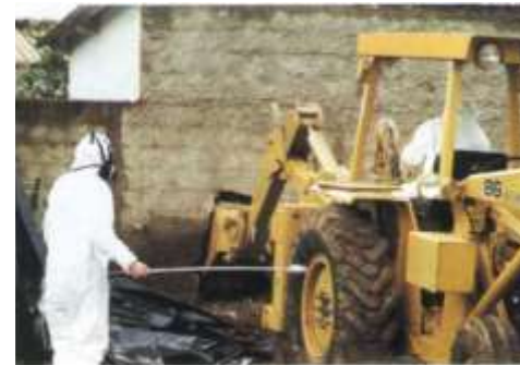
10. A hole is made to remove a radiation box upon giving a dose rate of 0.3 \text{ Sv h}^{-1} .
